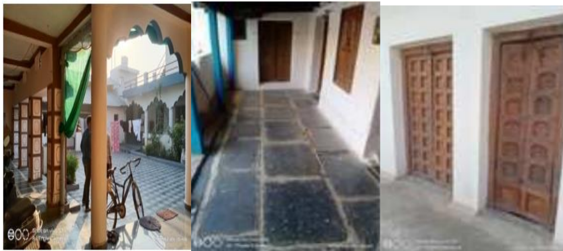
Figure 16. View of Courtyard, Slate Flooring, Multi panel door
