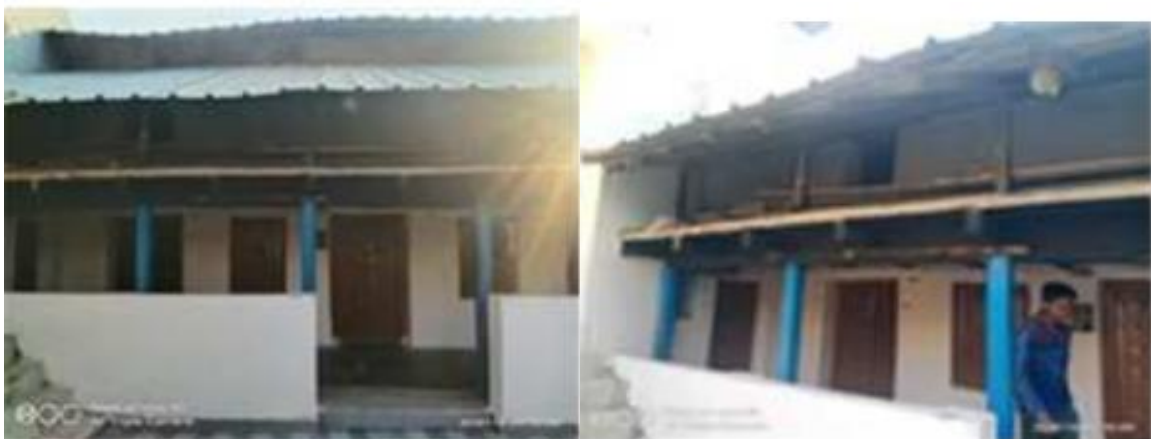
Figure 14. Shaded raised platform at the entrance, 2'0" high from road level.
