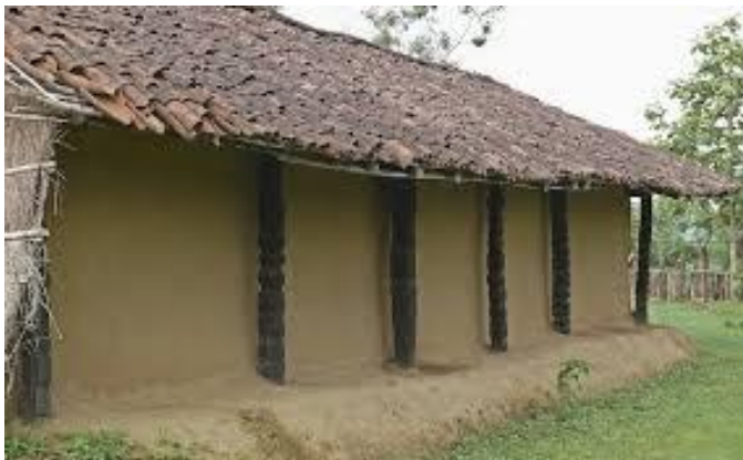
Figure 13. Tribal House architectural diversity.
