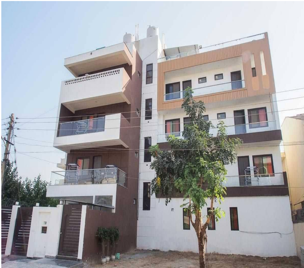
Figure 28. Exterior of PG Accommodation, Gurugram.
