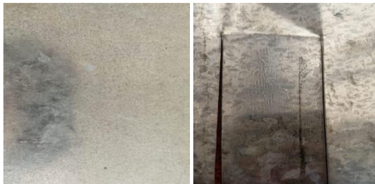
Figure 17. Before and after cutting the sheet metal respectively.
