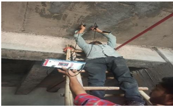
Figure 2. Rebound hammer test (RHT).
