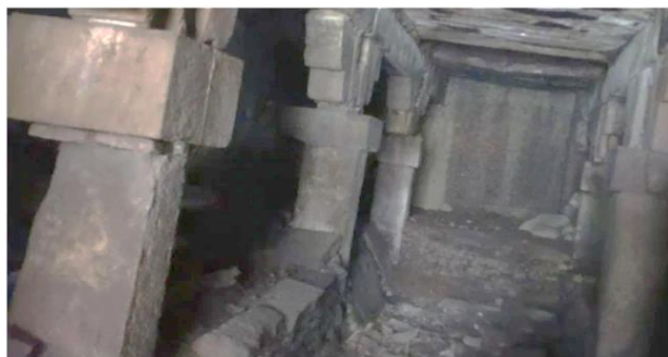
Figure 6. Reuse of the temple pillars to create a cellar to flatten the area at the front of Gyanwapi Mosque, to create a platform in 1792 CE (after India Today).
