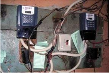
Figure 2. Injecting Foreign elements in the energy meter
