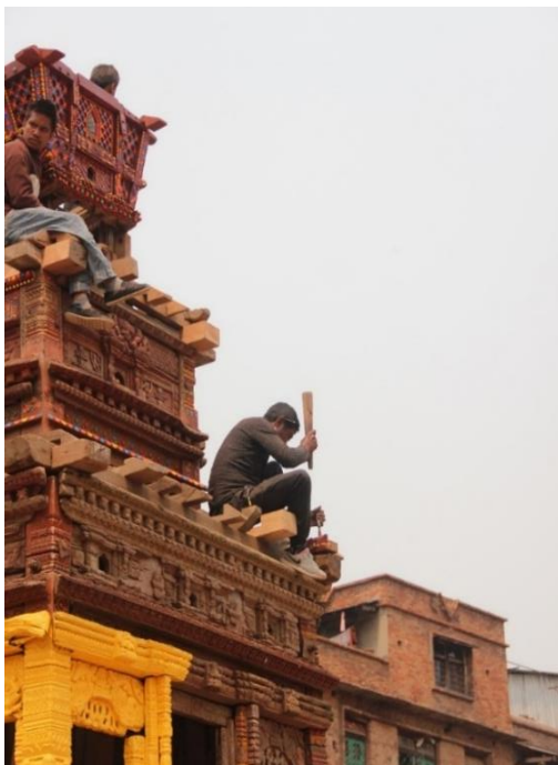
Figure 6. On-site alteration being done by the carpenters.
