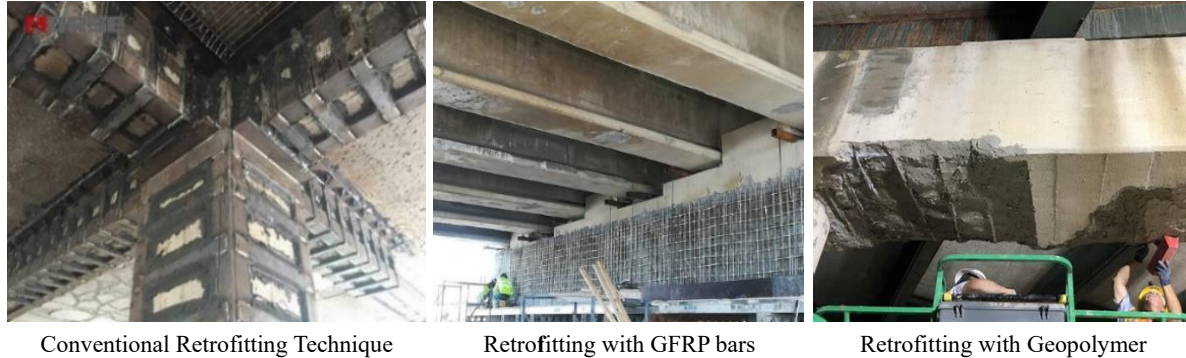
Figure 4. An illustration of retrofitting with various techniques.
