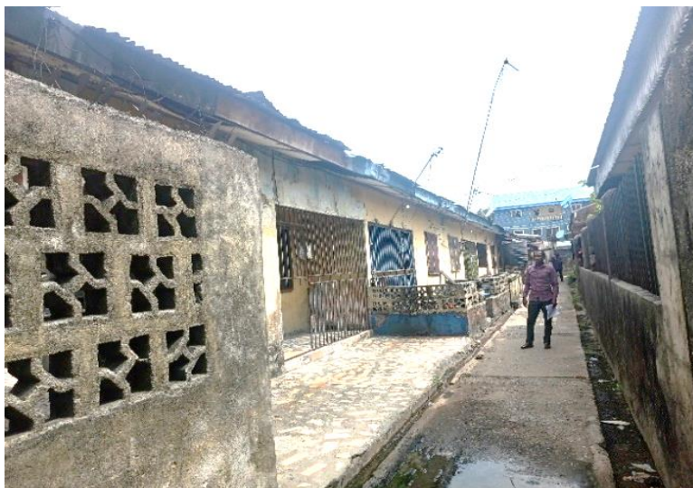
Figure 4. Building condition in study.
