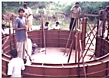
A. Steel shutter for Rammed earth wall
