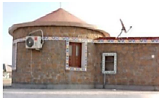
B. Using Air-Conditioning in Pacca Bhunga to Cool
