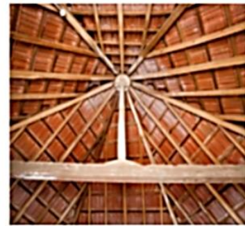
F. Mangolor tiles-roof interior details
