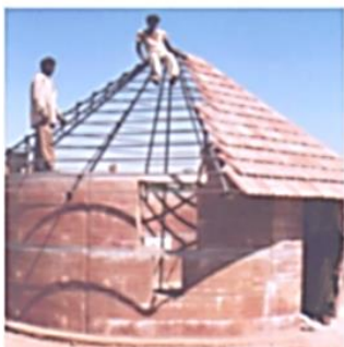
D. Hexagonal conical timber-roof
