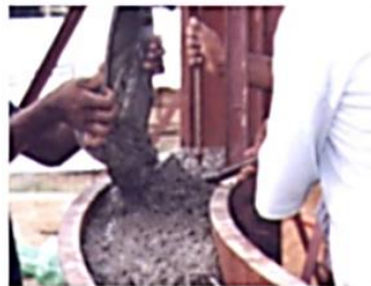
B. Filling the shutter with rammed earth
