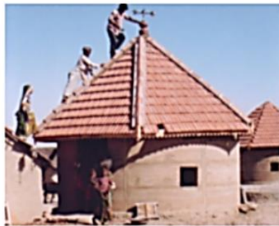
E. Hexagonal Mangolor tiles-roof finishing
