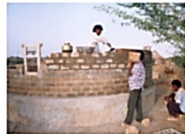
C. Brick wall on stone-masonry plinth
