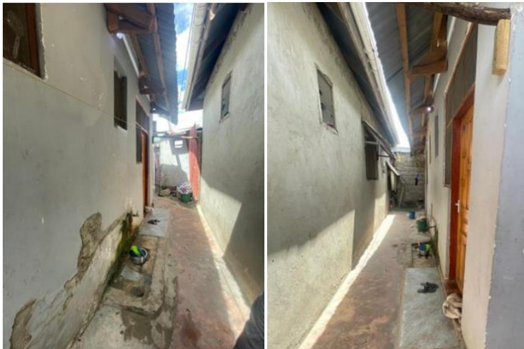
Figure 20. The narrow space between Case 6 House and the neighbouring building.
