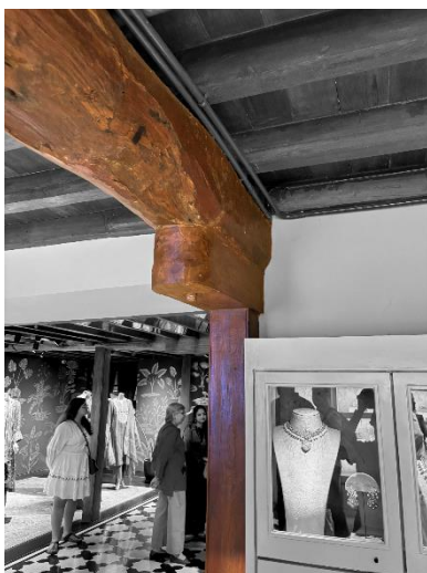
Figure 54. Exposed teak beams on the ground floor left uncarpentered and unpolished, to tell the story correctly.
