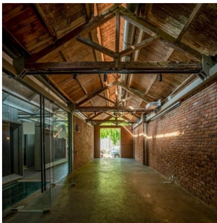
Figure 27. Substation after transformation.
