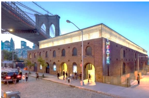
Figure 9. The transformation of the dilapidated shell into the St. Ann's Warehouse post adaptive reuse.
