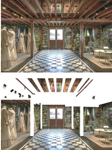
Figure 67. Imagined scenario of the ground floor with exposed teak members painted white to comply with regulations, resulting in a loss of spatial character.
