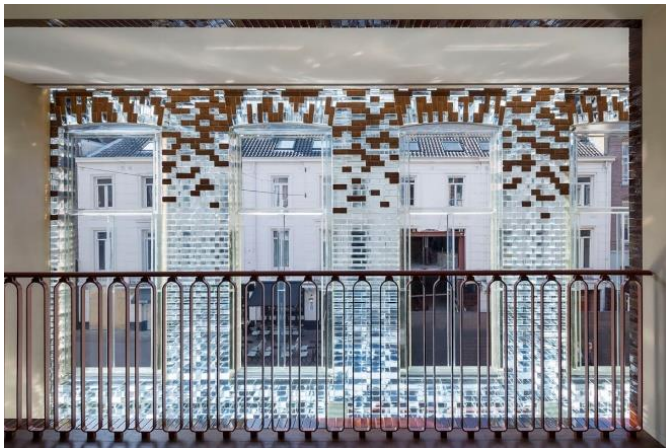
Figure 16. The seamless intersection between glass bricks and terracotta bricks as seen from the interior – showcasing the fusion of modern and traditional materials in the façade.
