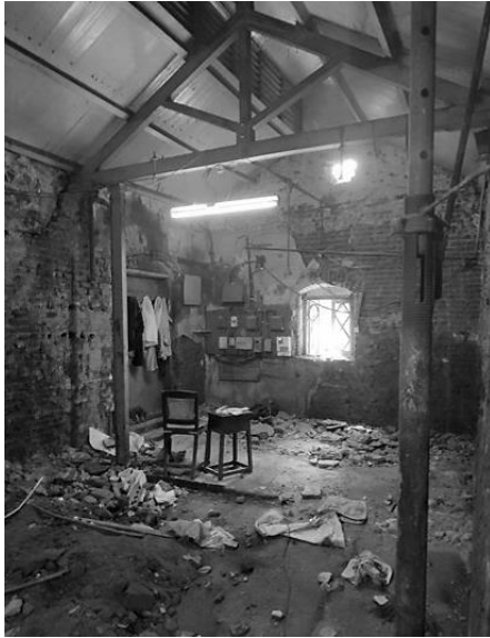
Figure 26. Substation before transformation.
