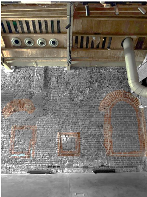
Figure 36. Remnants of the former industrial complex were preserved and revealed through the masonry wall of the ice factory. Air conditioning units have been inserted into the roof.
