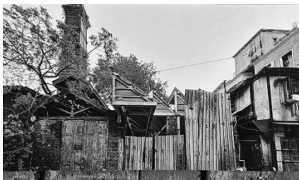
Figure 18. The dilapidated shell of the abandoned Ambico Ice Factory as seen during the process of adaptive reuse.
