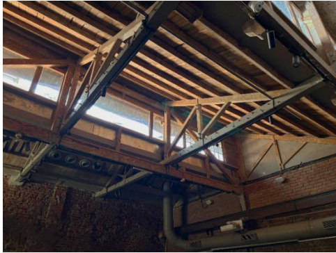
Figure 32. Visible wear, discoloration, and sagging timber roof members were intentionally retained and structurally reinforced with steel plates to preserve the industrial facility's historic character while ensuring structural integrity.
