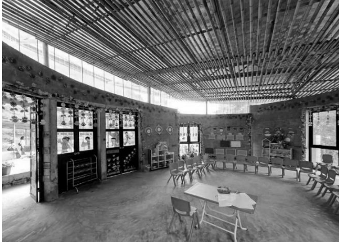
Figure 6. Interior view of classroom showing polycarbonate daylight band and bamboo ceiling.
