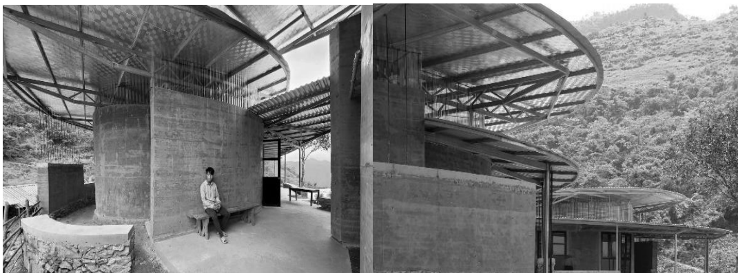
Figure 7. Rammed earth circulation spaces and sheltered walkways.
